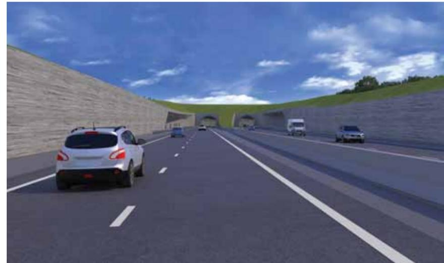
Figure 5.27: Driver's view of western tunnel entrance - vertical retaining walls option
