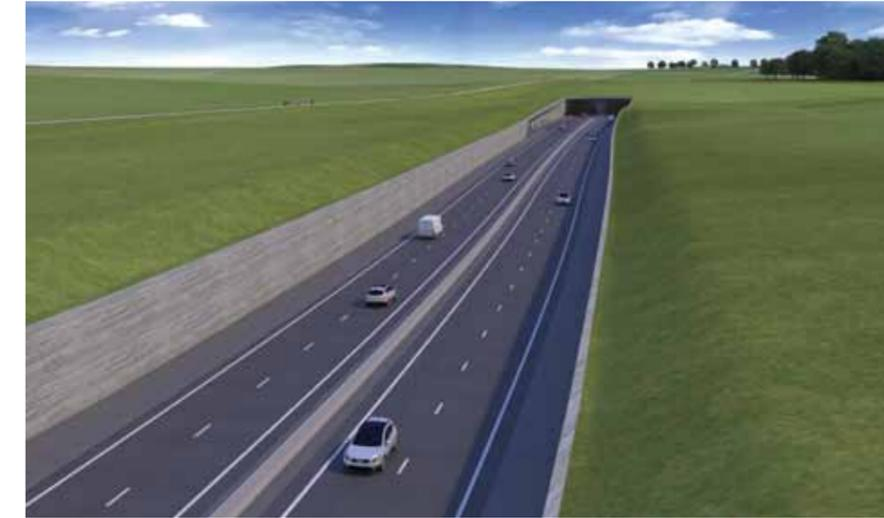
Figure 5.22: Approach option with vertical retaining walls
