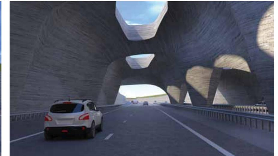
Figure 5.35: Driver's view of canopy with ventilation outlets - exiting
