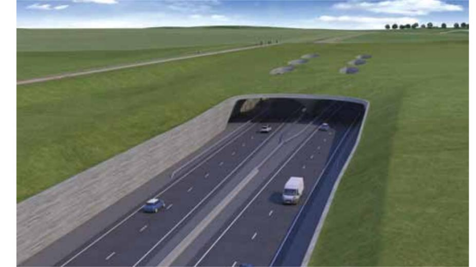
Figure 5.33: Grassed over canopy with ventilation outlets
